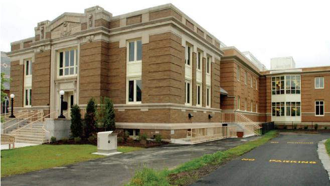
West Street view of the newly expanded & renovated library
